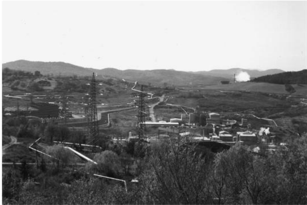
Fig. 4. Dry-steam plant, installations and transmission lines at Larderello (Italy) with a total exploited area of around 250 km 2 .
